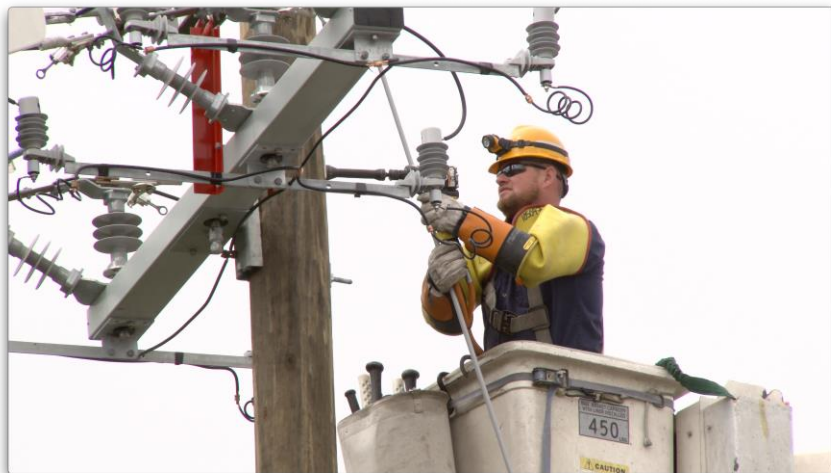
Figure 12: O&R Installing Distribution Automation Equipment
