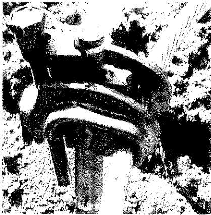
AMP WRENCH-LDC GROUND CONNECTION SEE NOTE 7
