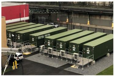
2 MW/10 MWh distributed battery system serving BQDM
