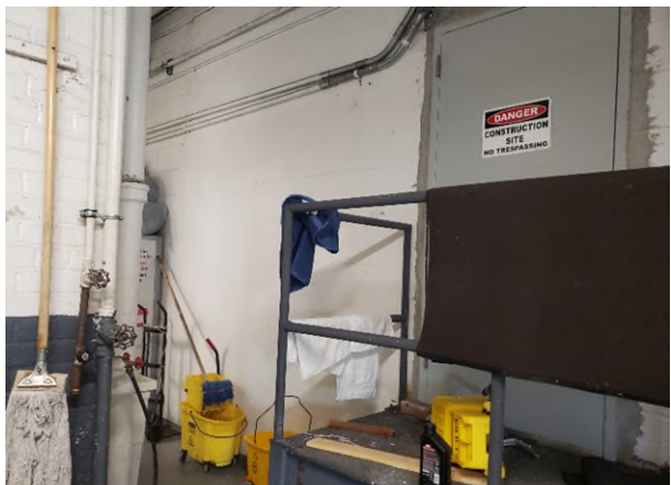
Photograph 12: Cleaning equipment in compactor room 20 feet from HPL-Compactor Rm air sample.
