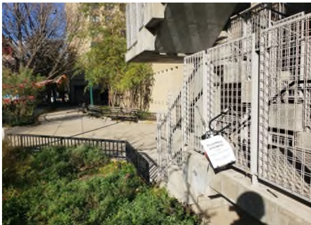
Photograph 5: AA-111820 air sample located on outside stairwell away from foot traffic and private driveway.
