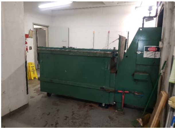
Photograph 9: Trash chute hopper in compactor room 8 feet from HPL-Compactor Rm sample.
