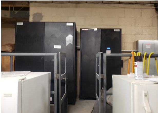
Photograph 14: Aerosol can in storage room in vicinity of HPL-Storage Rm air sample.
