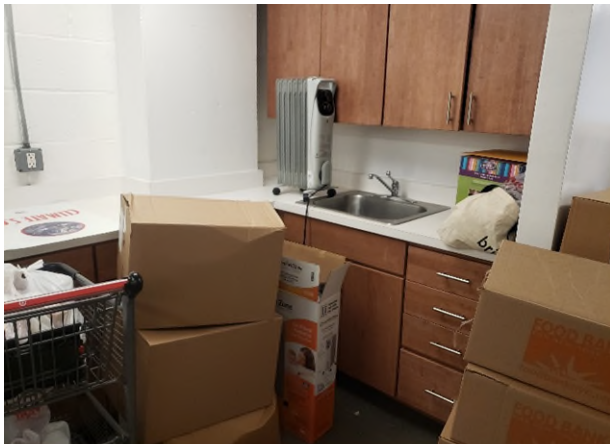
Photograph 31: Sink and space heater in vicinity of HPL-Meeting Rm air sample and DUP-111820 air sample.
