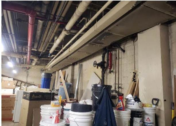
Photograph 20: Air duct running the length of the storage room ceiling.
