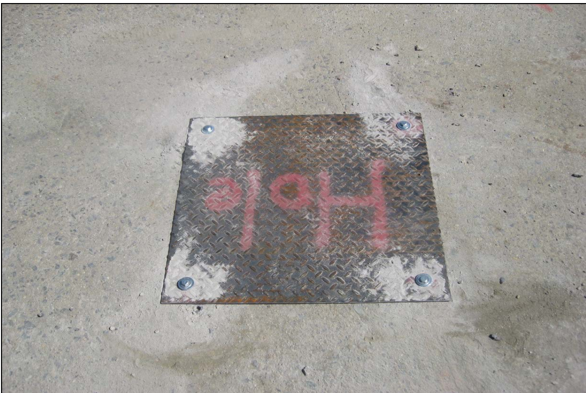
20. Steel plate installed over core hole and void at DB-2 location, 6/1/12.
