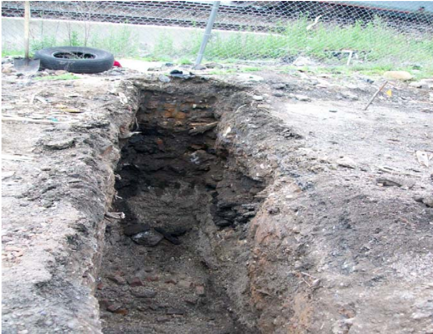
TP-1 at 8.5 ft bgs
