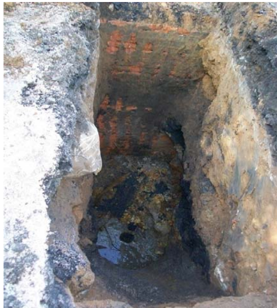
TP-5 to 9 ft bgs with holder wall reaching down to and passed water at 9 ft bgs
