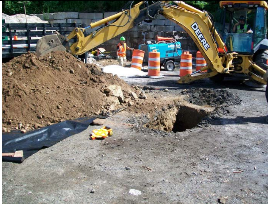
TP-3 and holder wall exposed at ~0.5 ft bgs
