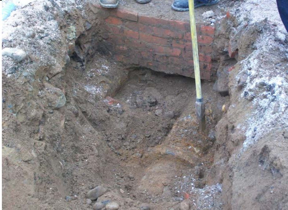
TP-4A and brick structure to the north with 2 ~12" pipes running southwest from under brick structure
