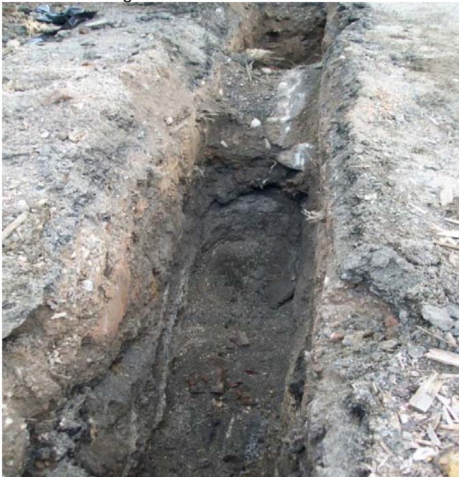
TP-1 Scraped holder bottom at 8.5 ft bgs
