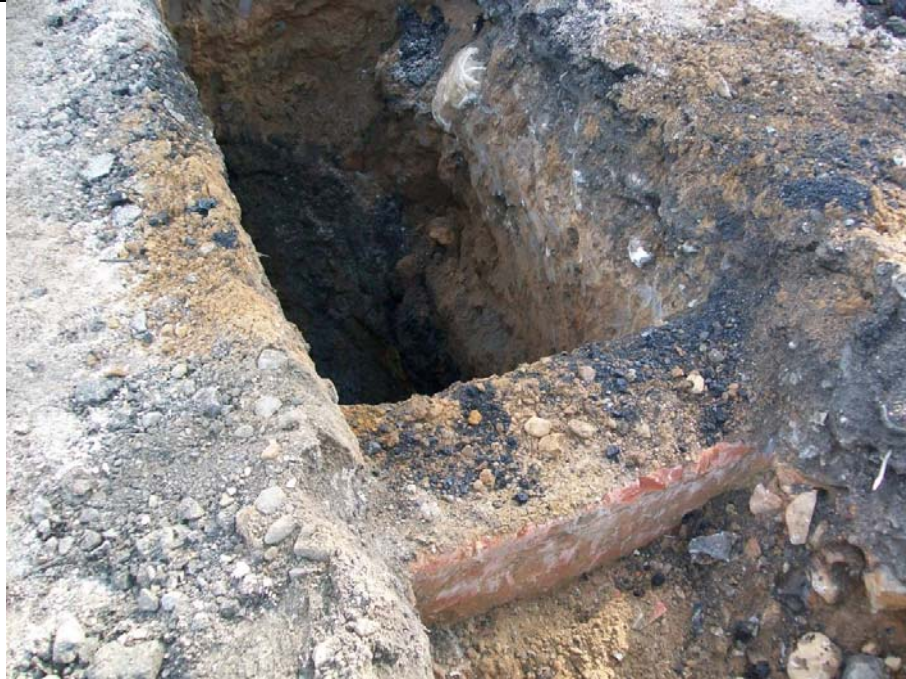
TP-5 to 9 ft bgs with holder wall in the foreground
