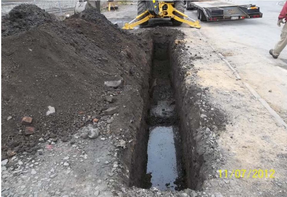
TP-6 at 6 ft bgs. Water intrusion at approximately 5.5 ft bgs
