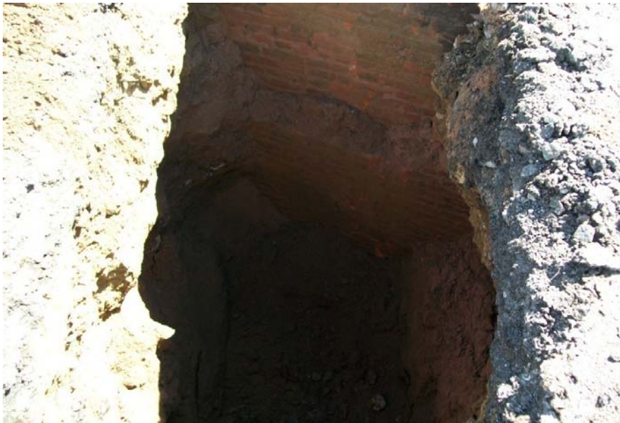
TP-3 and holder wall exposed to 9.5 ft bgs
