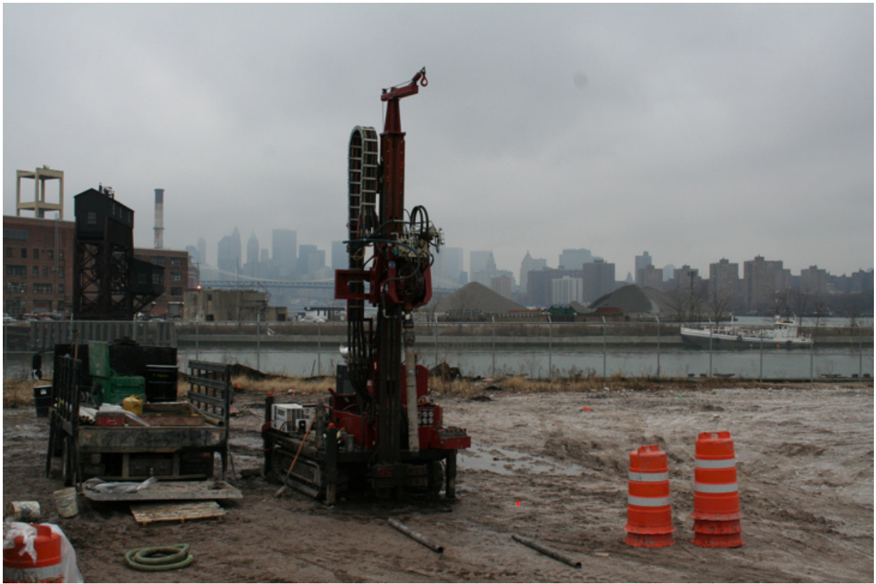
Photo 1: Roto Sonic Drill Rig and Support Truck.
