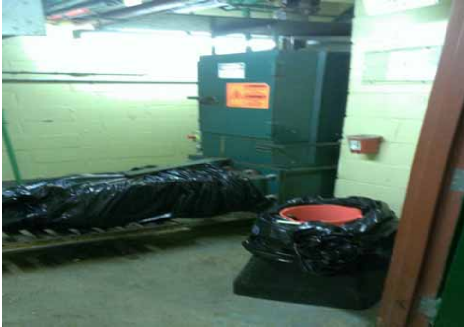
Compactor room (west) located within 1223 FDR Drive.
