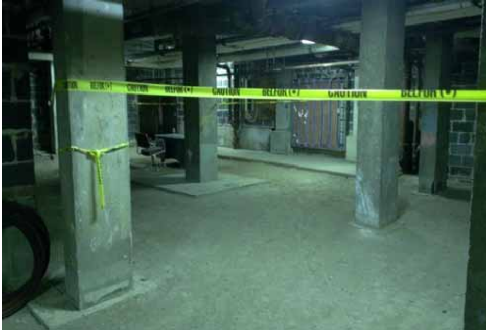
Entrance to tank room area (facing east) located in 170 Avenue D.
