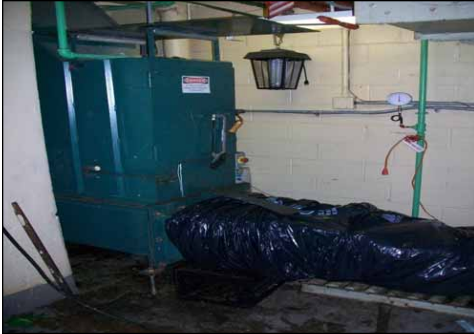
Trash compactor room (facing north) located within 1223 FDR Drive.
