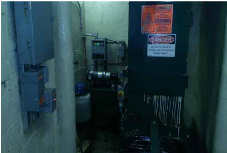
Compactor room (facing west) within 178 Avenue D.
