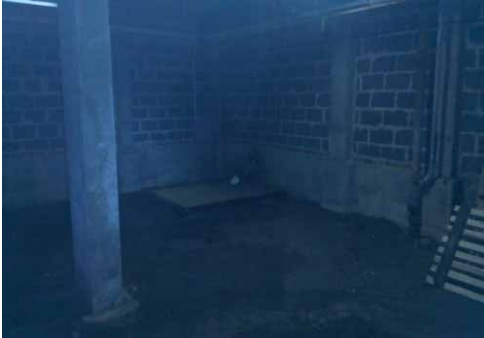
Storage room (facing south) containing various furniture located in 1223 FDR Drive.
