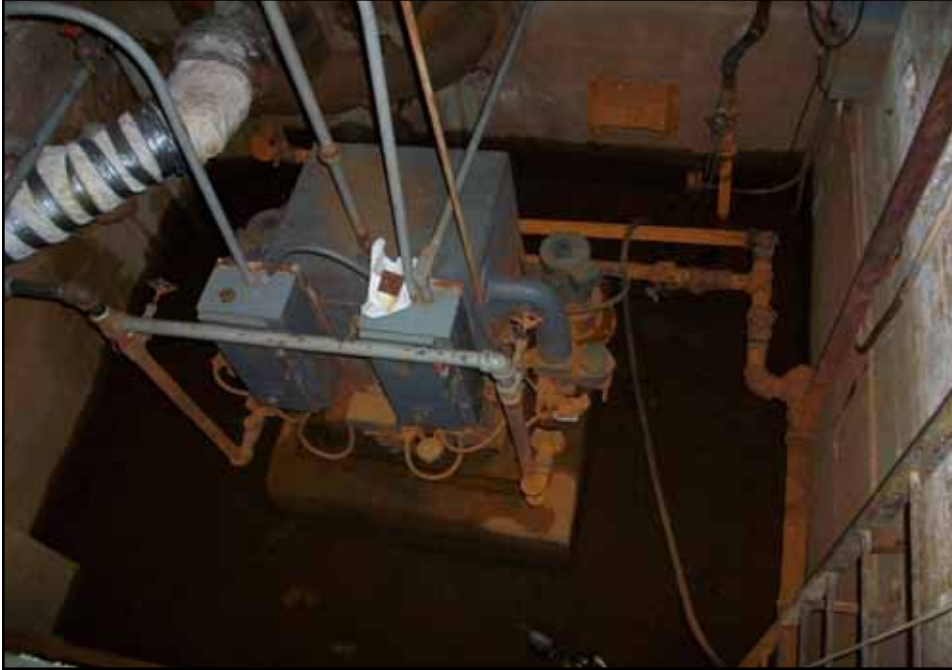
Pit containing sump in the tank room located within 1223 FDR Drive.
