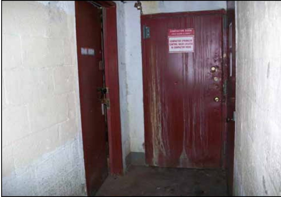
Hallway (facing south) containing tank room and compactor room at 1141 FDR Drive.
