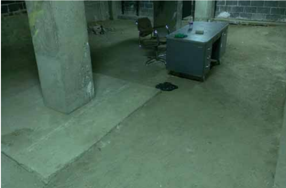
Miscellaneous storage near tank room facing east located within 170 Avenue D.
