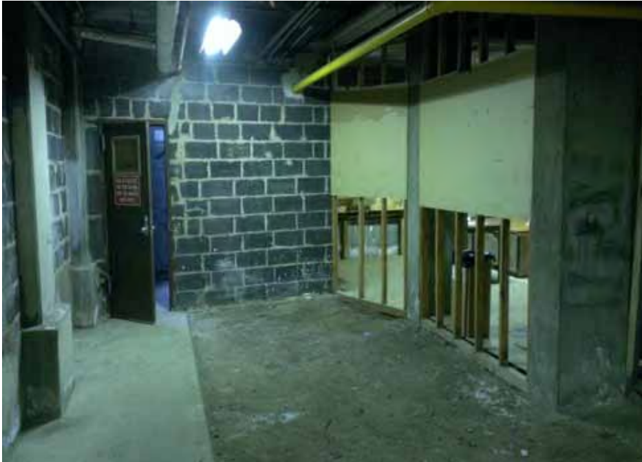
Storage room inside 170 Avenue D containing miscellaneous building materials.
