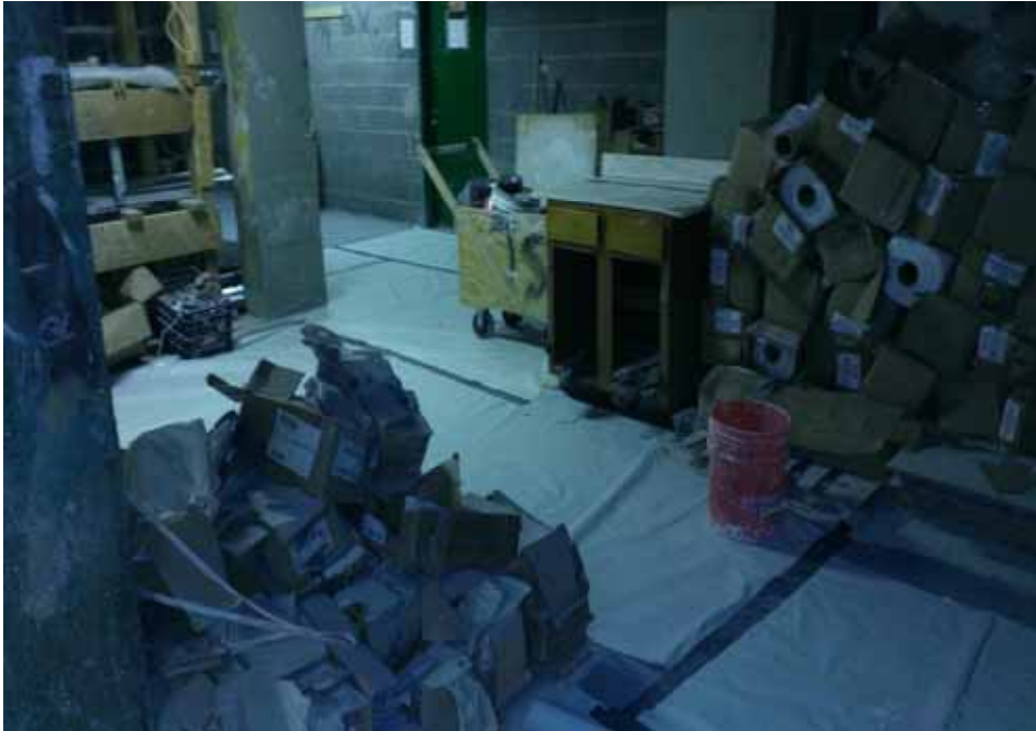
Miscellaneous plaster, tile, and adhesives located in plaster room (facing west) within 1115 FDR Drive.
