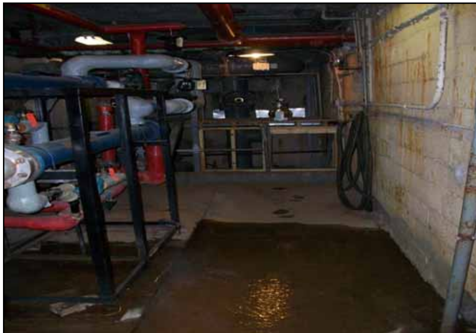
Tank room (containing JR-1115-IA- 3 (facing north) within 1115 FDR Drive. Two drains contained in floor with large fan and vents.
