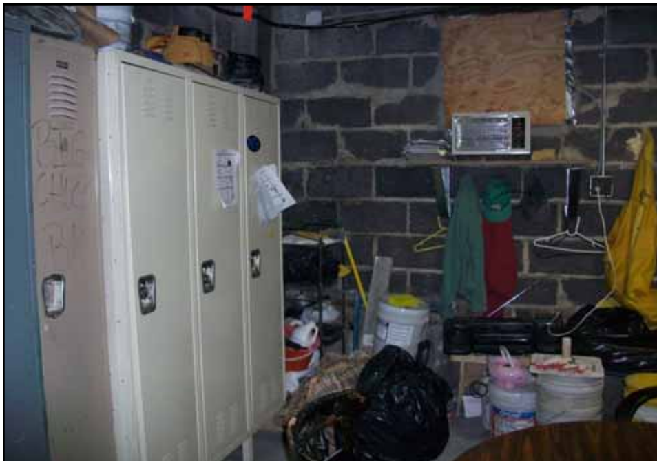
Various cleaning supplies and lockers (facing north) in plaster room within 1115 FDR Drive.
