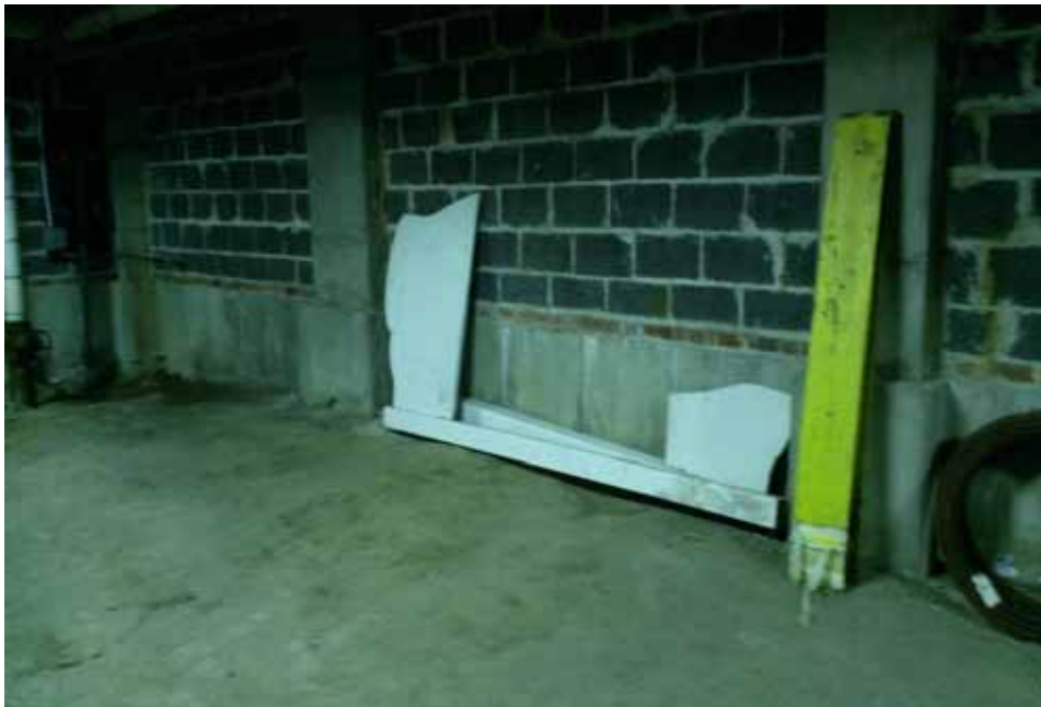
Entrance to storage room area (facing north) located in 170 Avenue D.
