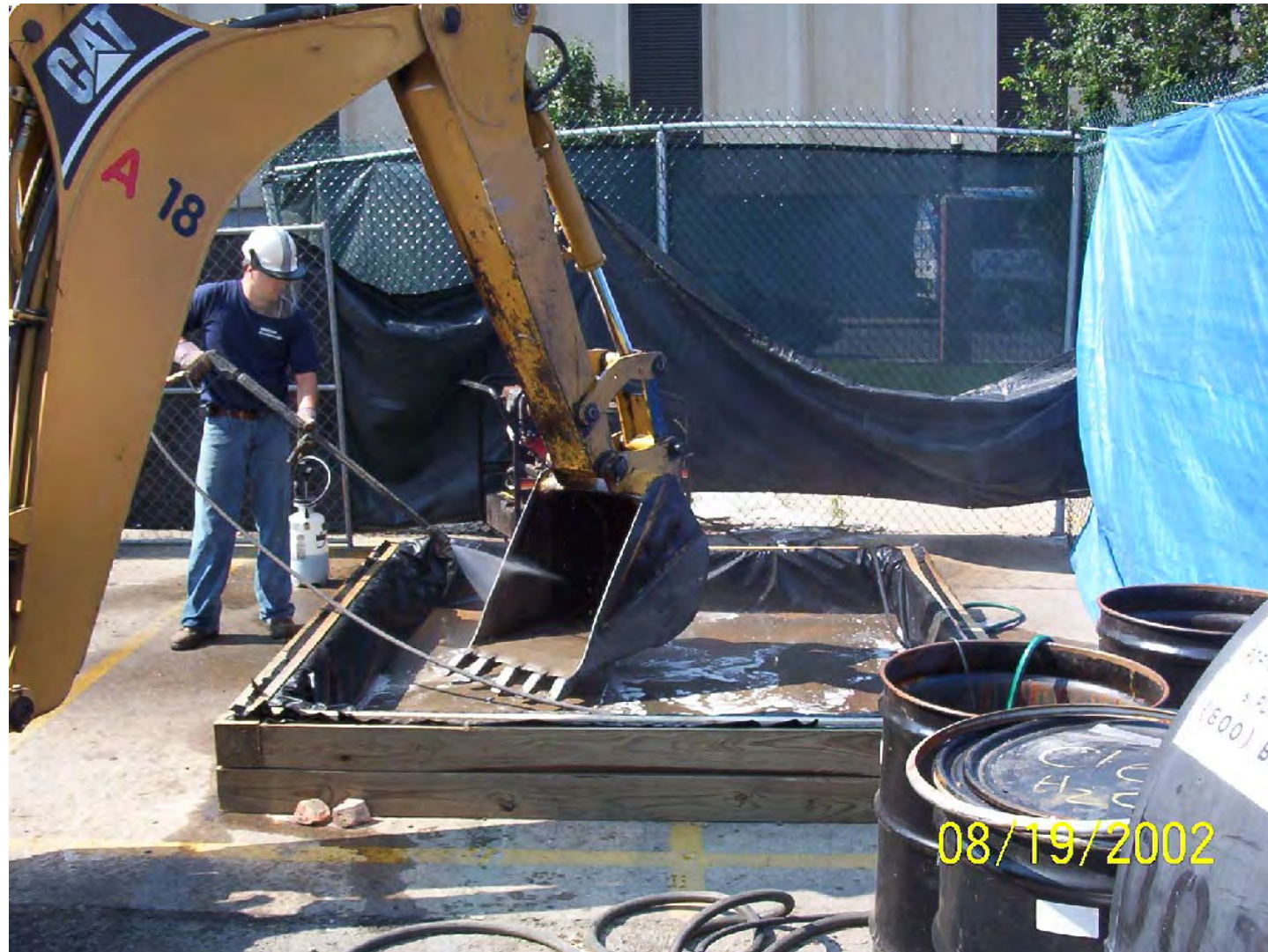
Decontamination procedures between test pits.
