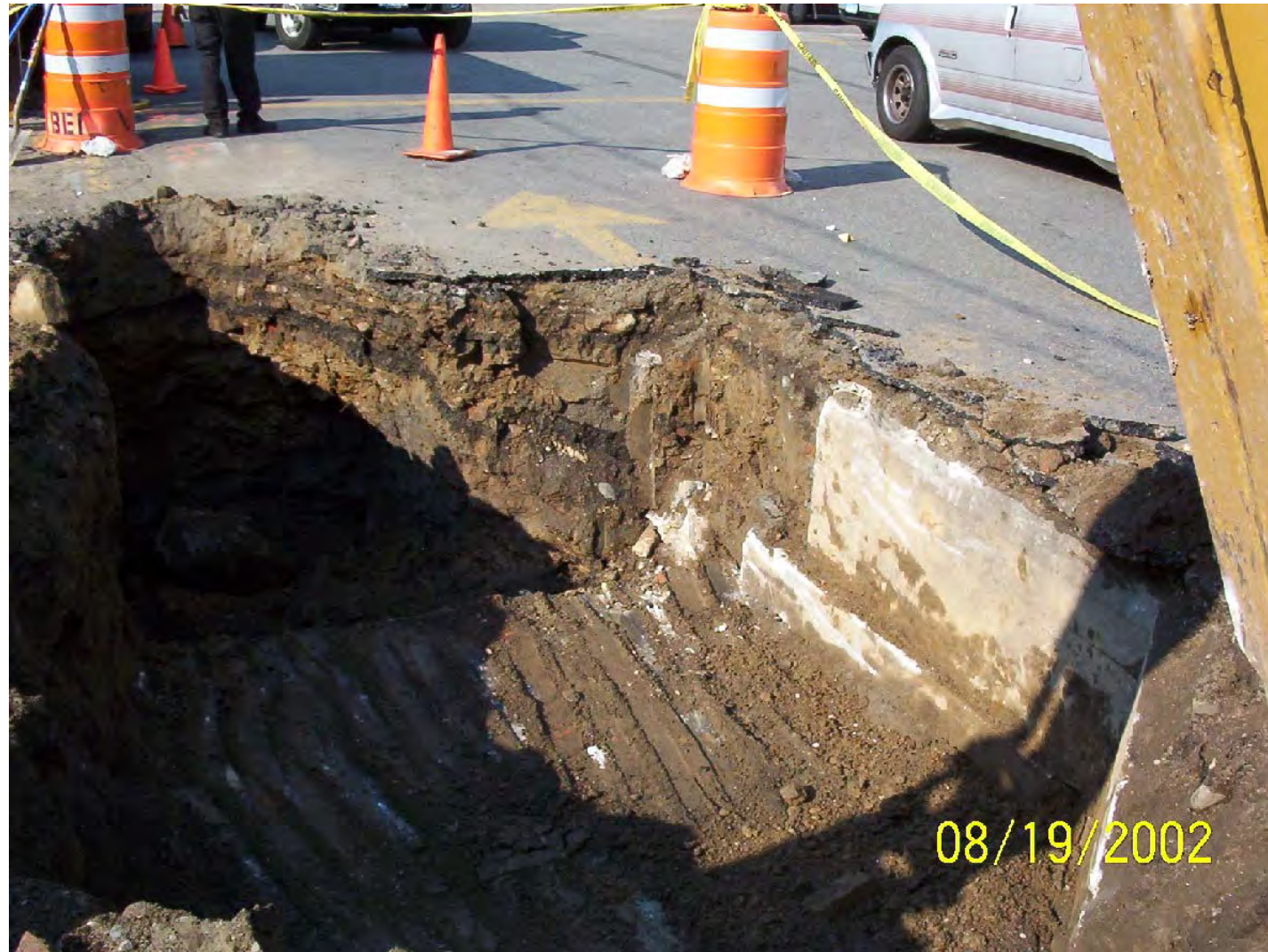
Excavated TP-03 to 11 feet below grade, looking southwest.
