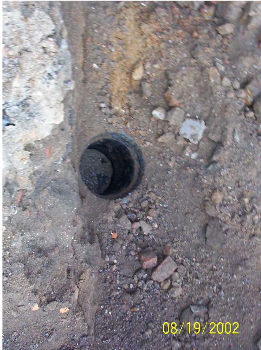
Main gas pipe encountered in TP-07.
