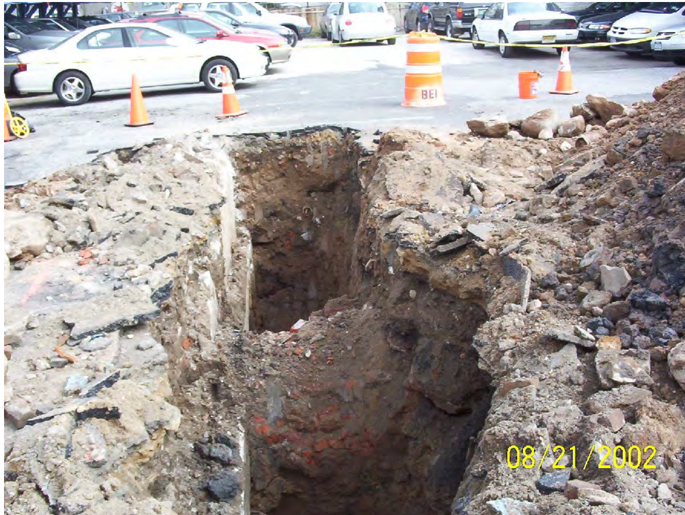
Gas holder brick wall encountered in TP-08, looking north.
