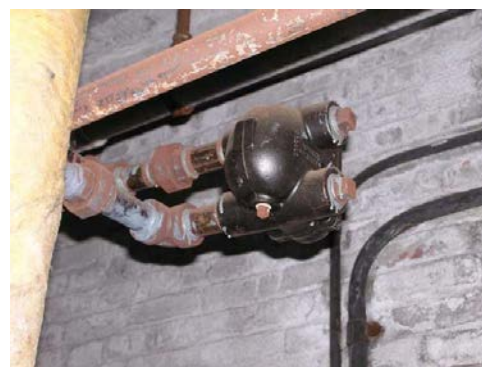
Figures 15 & 16: Main steam traps should be inspected as often as is recommended by the trap manufacturer.
