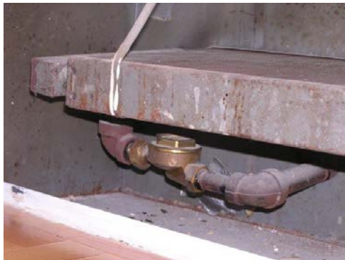
Figure 14: Radiator steam traps, such as this one, should be inspected at intervals recommended by the manufacturer.
